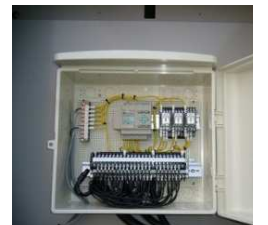
Automatic control system of air-conditioners
