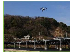
Drone IR inspection
