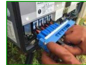
I-V characteristic inspection
