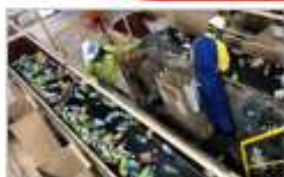
Waste separation equipment (equipment for recycling)
